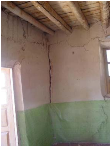
Figure 23a: Typical external walls damage in Firoozabad-Kagoor earthquakes [3]
