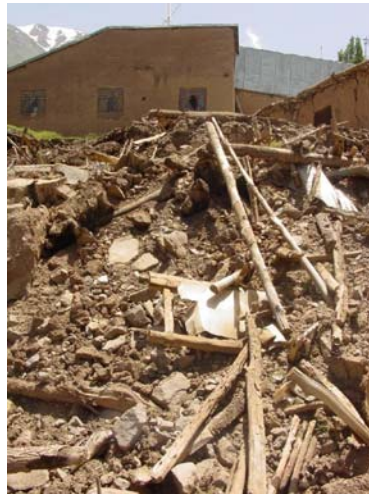
Figure 27: Total collapse of stonework building in Firoozabad-Kagoor earthquakes [3]
