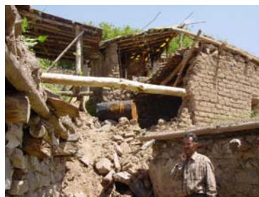
Figure 25: Typical roof damage in Firoozabad-Kagoor earthquakes [3]
