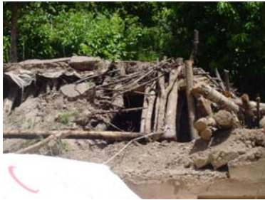
Figure 26b: Typical roof damage in Firoozabad-Kagoor earthquakes [3]
