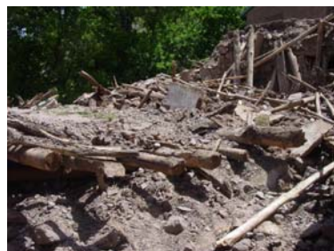
Figure 26a: Typical roof damage in Firoozabad-Kagoor earthquakes [3]
