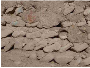
Figure 2b: Typical Building Wall View [3]
